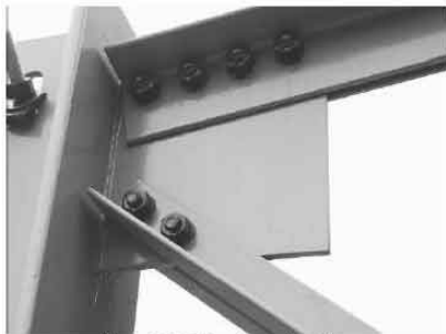
Figure 7-17. Misc. Connection: Truss Column C2 / Truss B7
