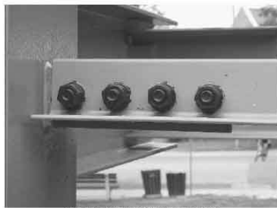
Figure 7-18. Misc. Connection: Truss Column C2 / Truss B7
